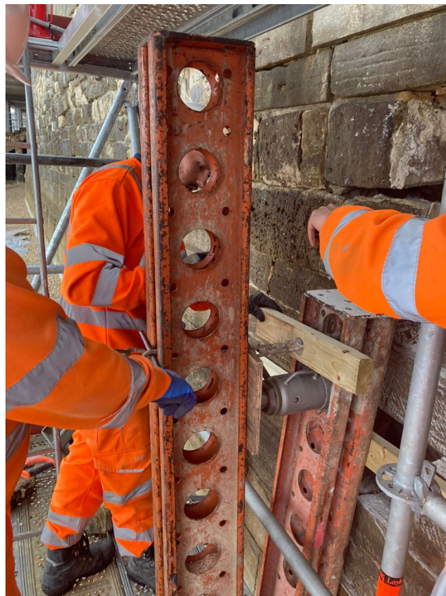
Figure 2: The original blocks that had been retrieved from the foreshore being reset in their original position
